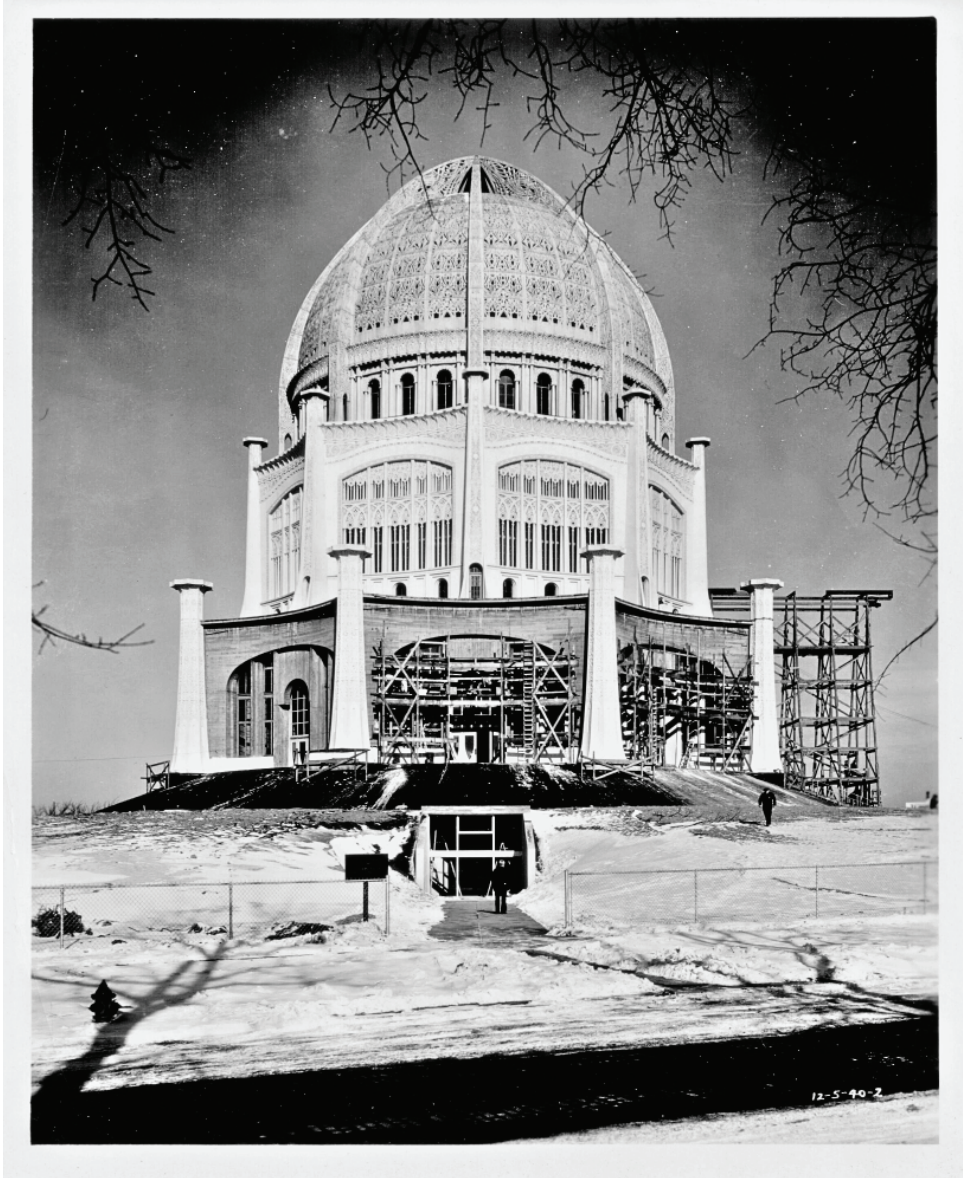
5 December 1940, Main structure approaches completion, Bahá'í House of Worship, Wilmette, Illinois
